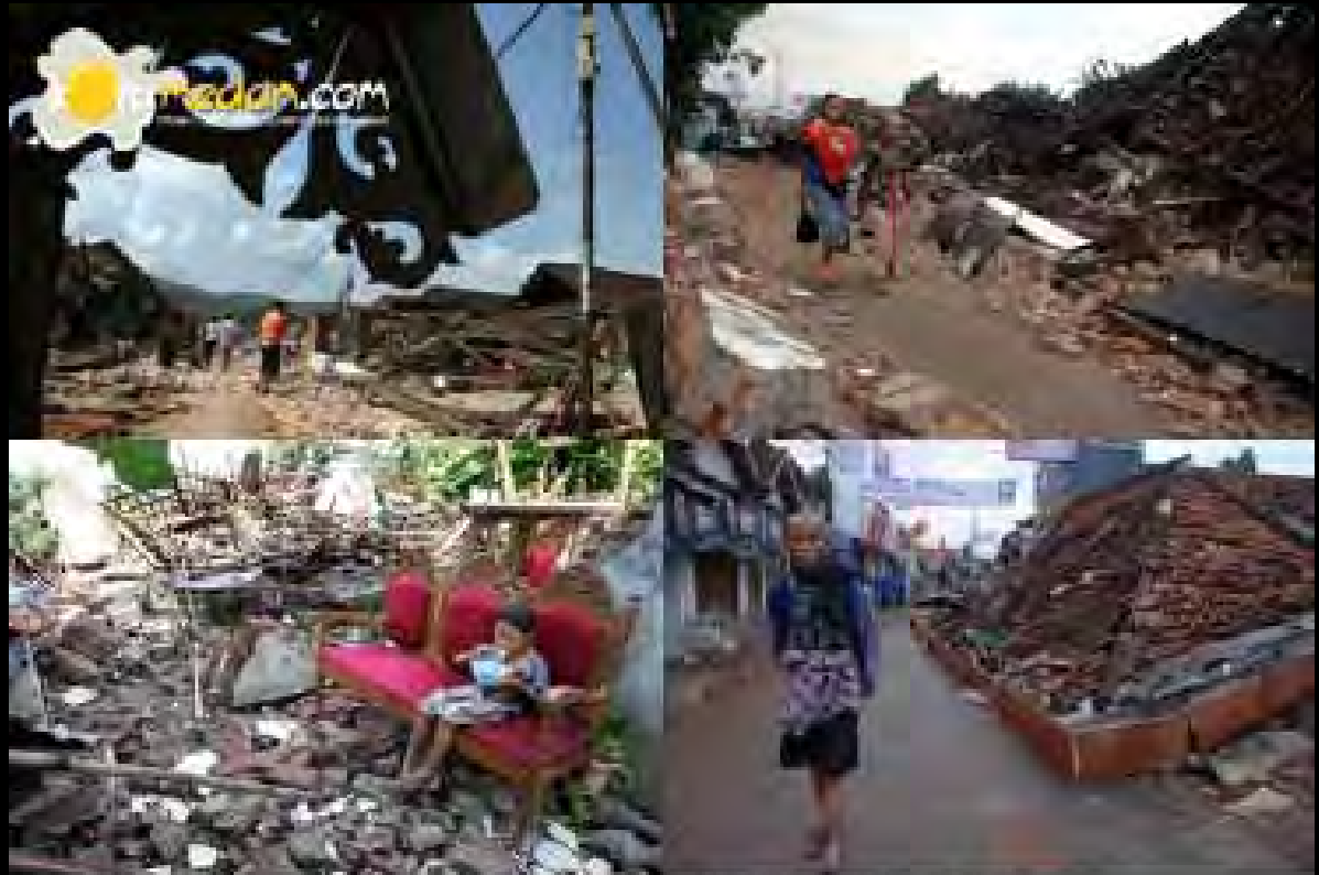
Destroyed houses at Bantul, Indonesia caused by 6.2 magnitude earthquake on Java island
